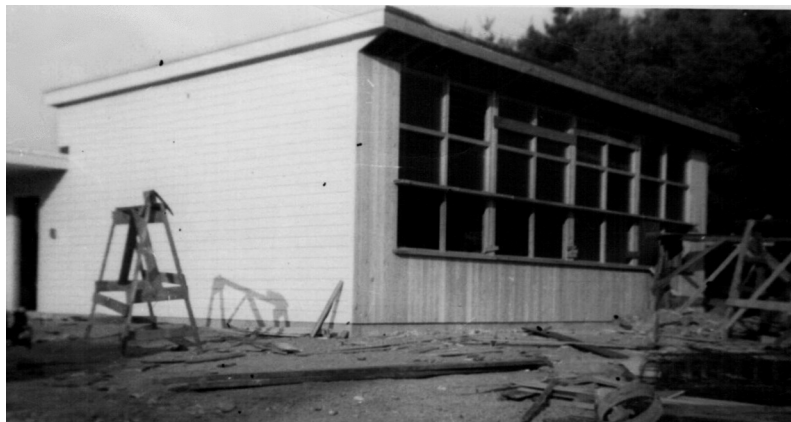
1 st Grade classroom under construction 1951
