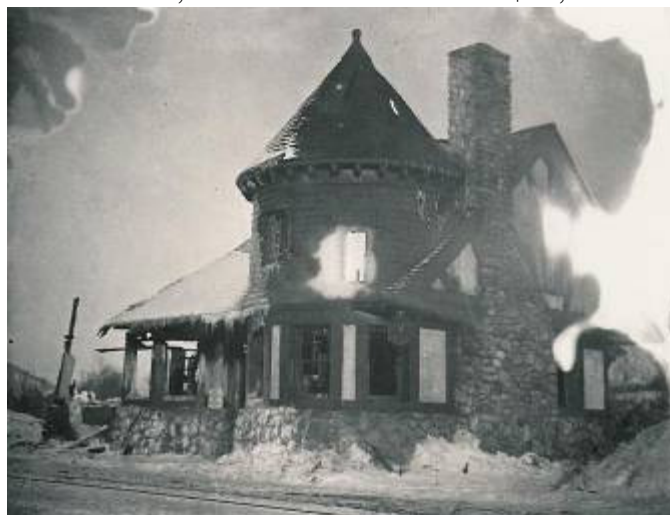
Damage to the photograph makes the Depot look like it's still on fire.
