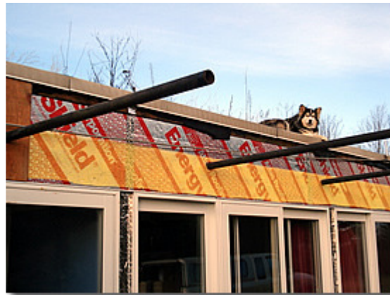
Duke supervises construction
